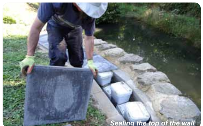
The wall takes shape ...
