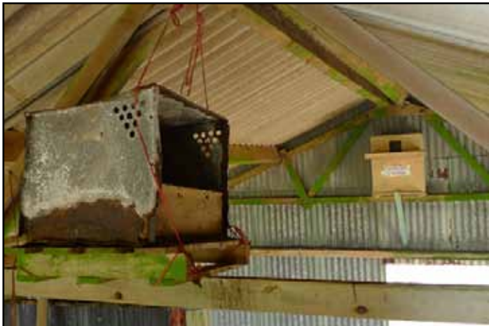
The new box is placed higher than the old one which will be removed once the owls have started using the replacement
