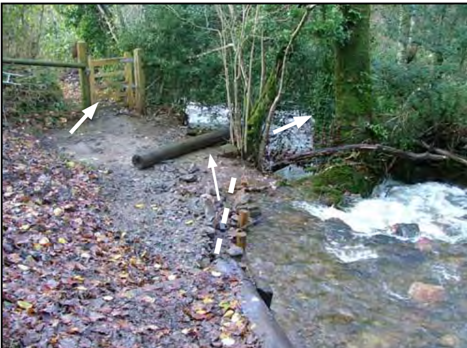
The water was far higher than we'd ever seen it before - the arrows show where the water reached and the dotted line where the pole was Photo: Frances Ramsden
