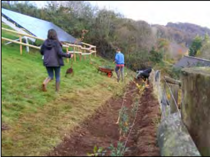
Hungarian trainees on placement in November plant the new hedge below the solar panels Photo: Matthew Twiggs
