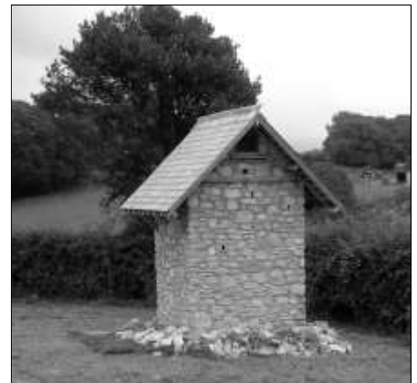
Before the final touches were made David (BOT) and presenters Jem (2nd left), Bill and Dusty (right) posed for this picture - note the skip still in the background. Stone piles were left at the foot of the
