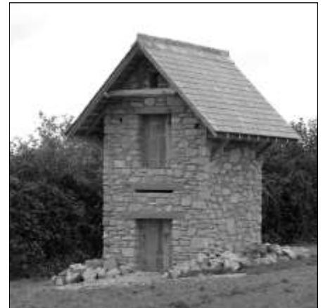
refuge to provide a habitat for amphibians and reptiles. From this side you can see the provision for kestrels and holes for little owls, sparrows and other birds. On this side there is access for Barn Owls,
